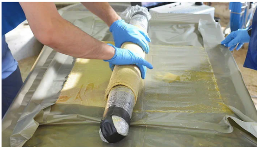
Trelleborg DrainPacker Training at SECA
