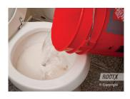
to push foam down the toilet drain. To avoid overflow, use no more than 908g jar of RootX for toilet application.
