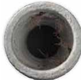
With RootX, debris is decaying and roots are stunted.
